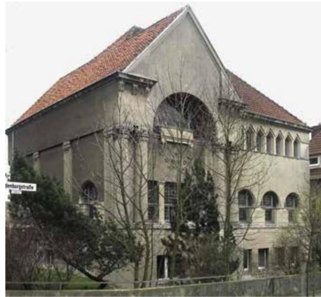
Peine, Lessing Lodge, east facade. Representative design of the facade by changing the surface arrangement; (blue): scratched plaster; (yellow): cast concrete plaster, dressed by a stone mason using a charring chisel; (green): dressed concrete, partly prefabricated before transferring it to site. Photo / graphic: HAWK / Götz, 2007.
