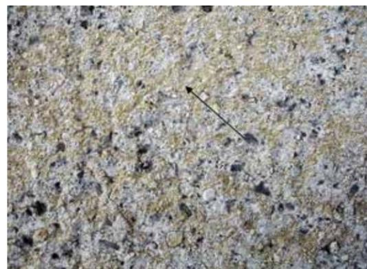
Peine, Lessing Lodge, east facade, scratched plaster, detail of the cleaned surface. Through the cleaning, the weathered structure and yellowish discoloration of the surface became apparent. Photo: HAWK / Götz, 2007.
