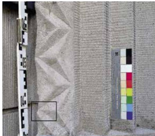
Peine, Lessing Lodge, west facade, entrance area / stucco edging. Condition after the repair. The repair plaster adapted very well in color and structure to the original material.
