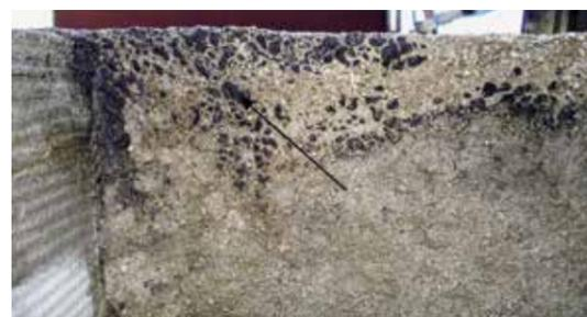
Peine, Lessing Lodge, east facade, basement, detail, surface of the lintel. Crusting and blackening in the edge areas despite cleaning twice. Photo: HAWK / Götz, 2007.
