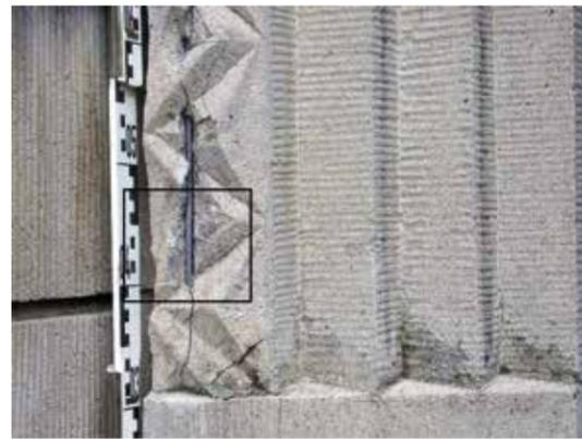
Peine, Lessing Lodge, west facade, entrance area / stucco edging. Damage in the cast stone. The corrosion products on the iron reinforcement were removed with the sandblaster.
