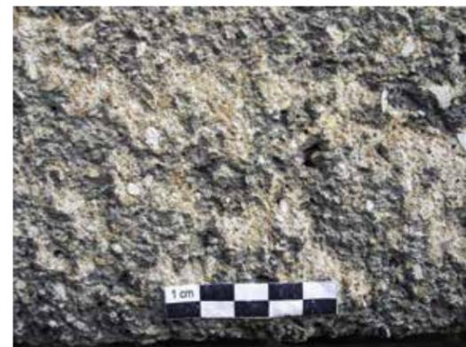
Peine, Lessing Lodge, east facade, base, detailed view: cast concrete plaster with horizontal joints and dressed treatment by chisel. Photo: HAWK / Götz 2007.
