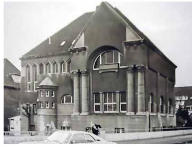
Peine, Lessing Lodge: The two pictures from 1973 show the north and west (left) and east façade (right). The surfaces are very dirty. Signs of weathering can be clearly seen on the scratch plaster and plinth surfaces.
