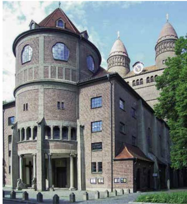
Ulm, ev. Paulus church, 1908-1910, according to plans by Theodor Fischer. Facade with pre-mixed concrete: trickled concrete (cement, sand, bean gravel 1:1:2), processed with two-pointed edge. Photo: Density, 2007, wikimedia commons.
